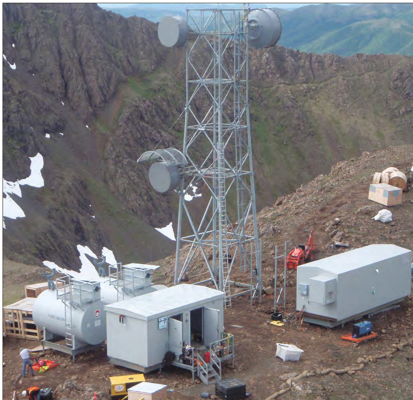
This view shows work under way at the Kulukak Mountain site.
